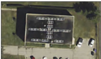
Image 1 - The solar panels from an aerial photo.
